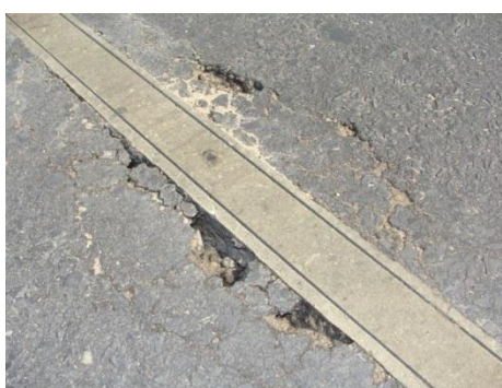
Figure 8 – Pavement deterioration of MS-WIM site
